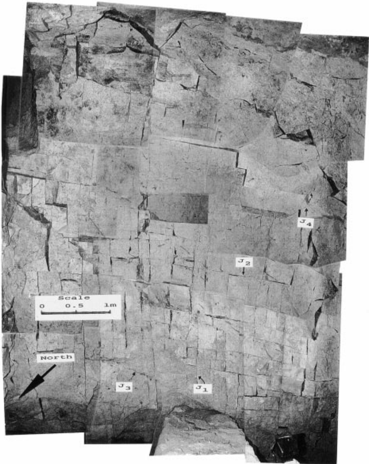
Fig. 4. Photograph collage showing the roof of room 1. The prismatic blocks are formed by members of joint sets 1 and 2 with mean joint spacing of 20 and 25 cm, respectively. The horizontal bed thickness is about 50 cm.
