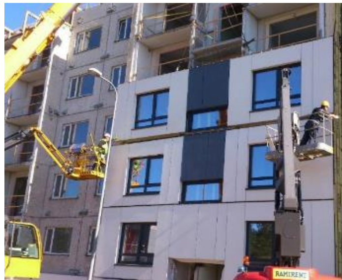
H2020 MORE-CONNECT pilot Tallinn, Estonia: Large and heavy boards are very demanding to install
