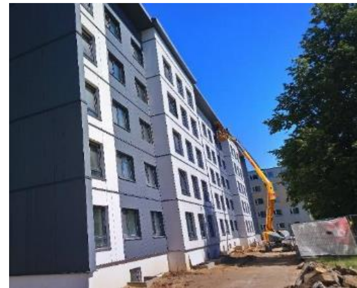
H2020 MORE-CONNECT pilot Tallinn, Estonia: Large and heavy boards are very demanding to install
