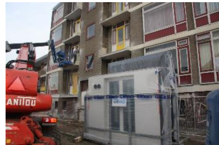
H2020 MORE-CONNECT pilot Arnhem, The Netherlands: Smaller and lighter boards, easier to handle
