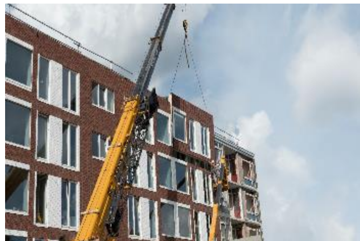
H2020 MORE-CONNECT pilot Arnhem, The Netherlands: Smaller and lighter boards, easier to handle
