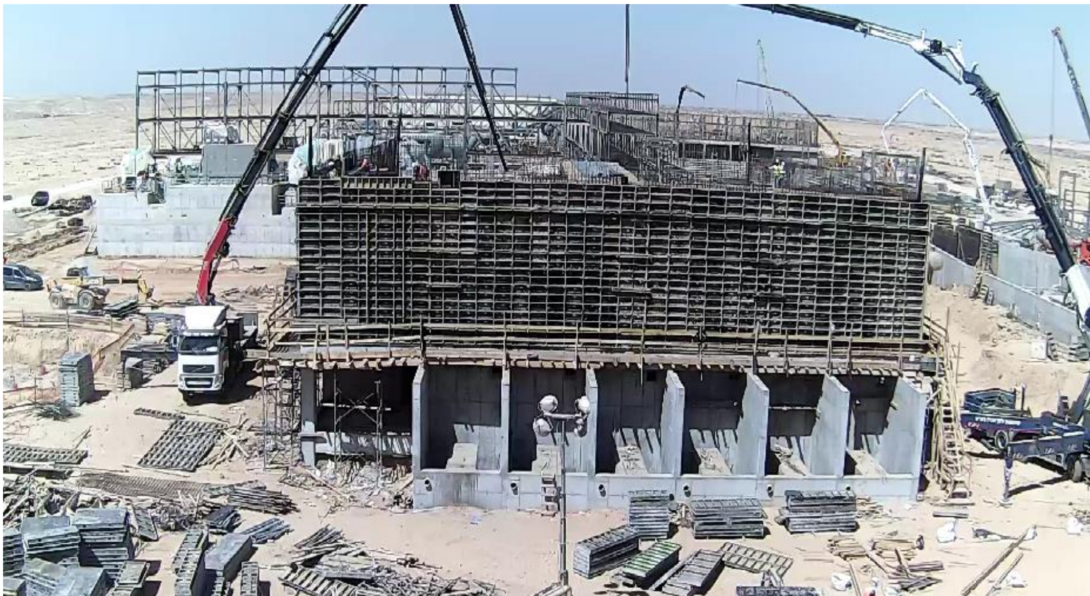
Construction - Main Electrical Building civil works
