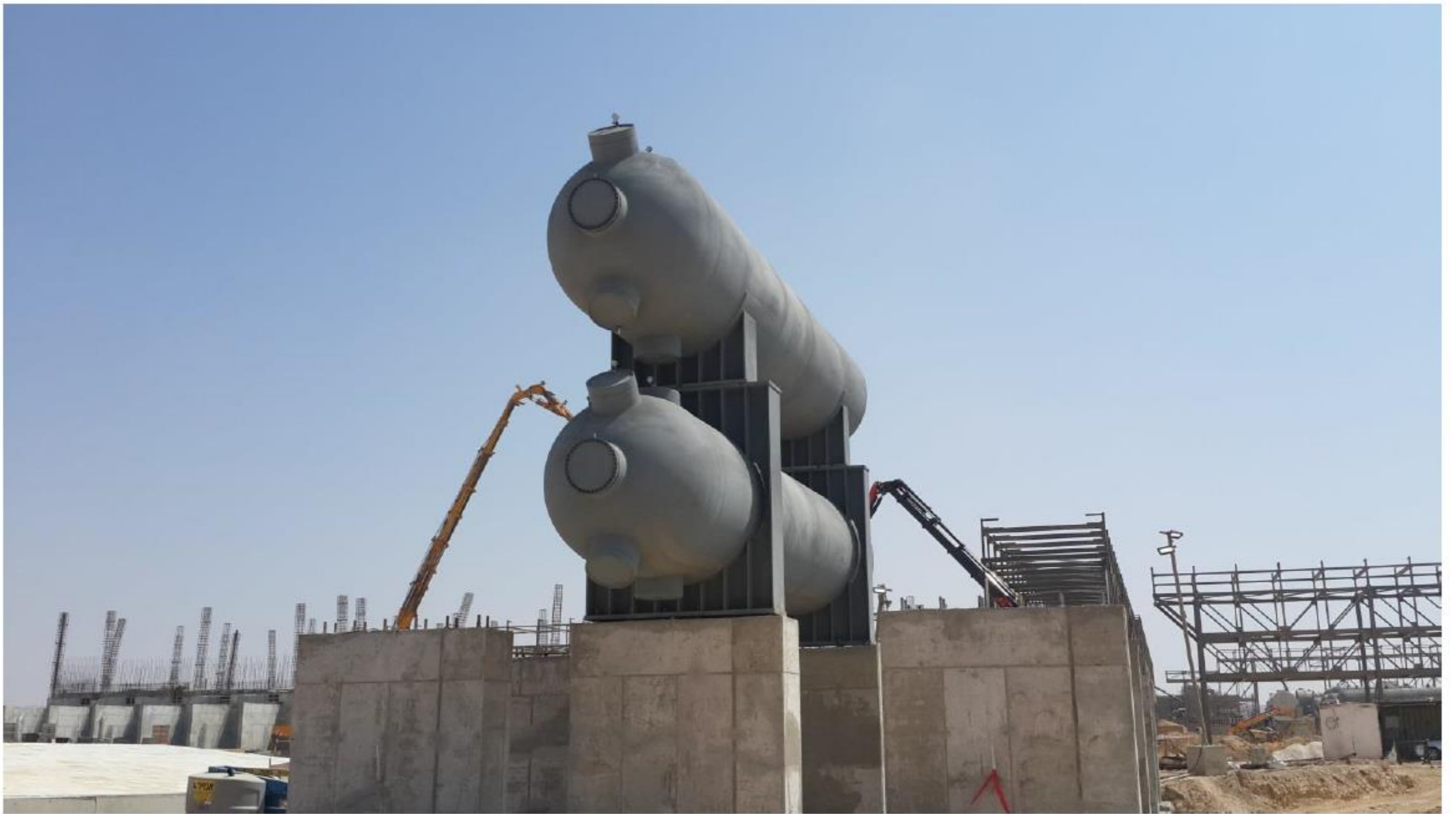
First Pair of TES Heat Exchangers Erected
