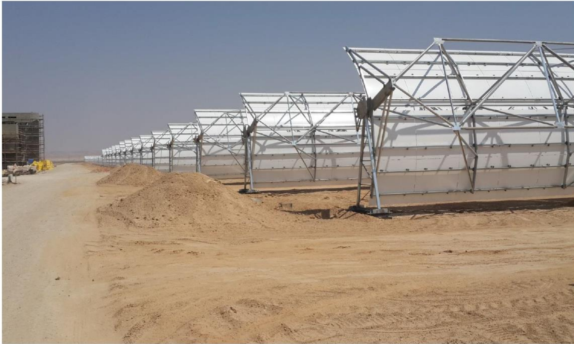
New Mirror Modules Erected in Area 4
