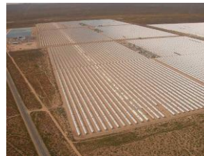
SEGS, 1980's 9 trough plants 354 MW e , CA
