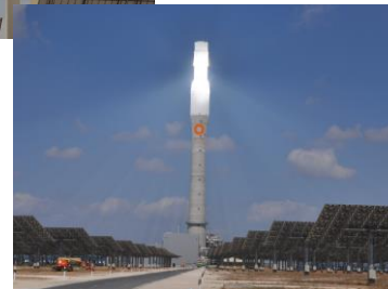
Gemasolar, molten salt, 19 MW e , Spain, 2011
