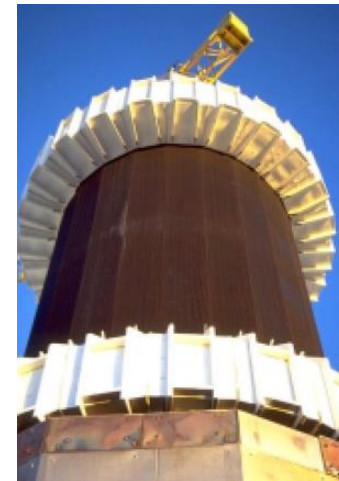
External tubular receiver
