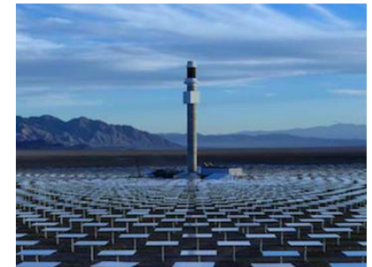
Crescent Dunes, molten salt, 110 MW e , NV, 2015
