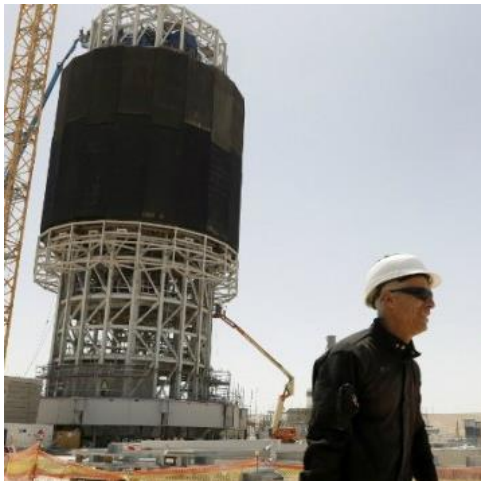
Receiver and heliostat field under construction
