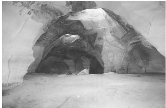
Fig. 2. Set of caverns with overlapping volumes, the width of the caverns varies between 20–25 m.
