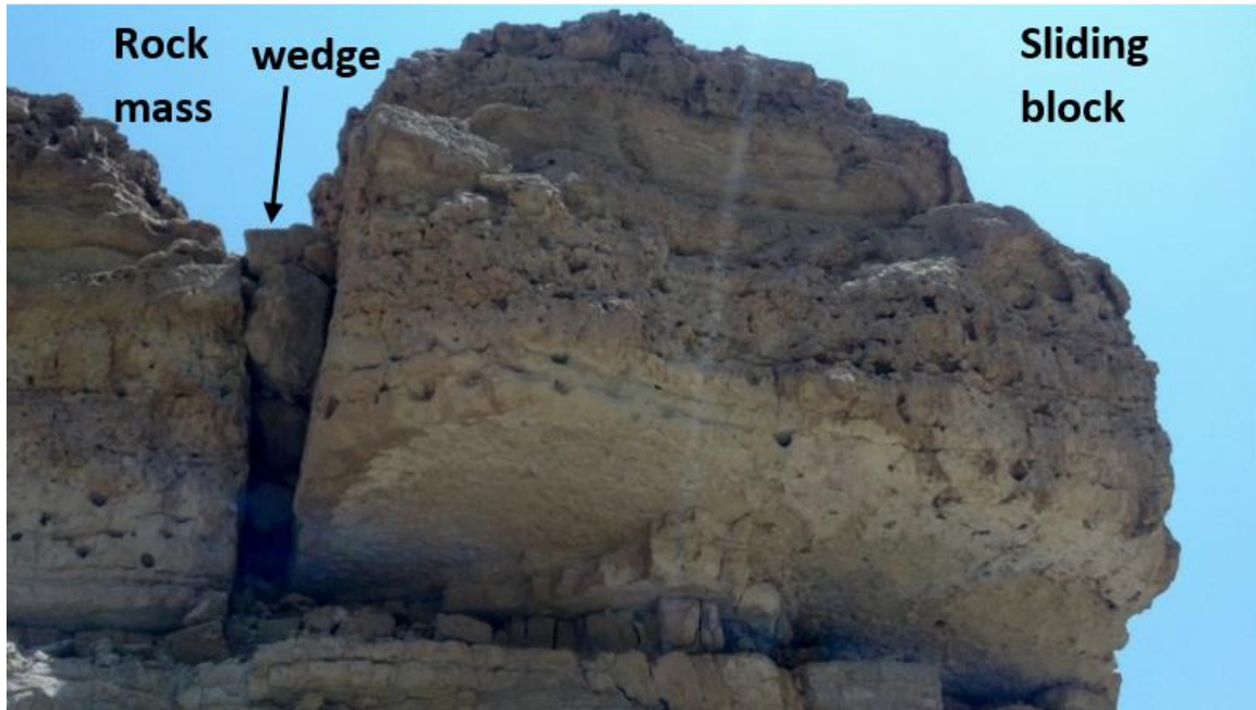
Figure 1.5 - Wedge inside a tension crack, Wadi Arugot
