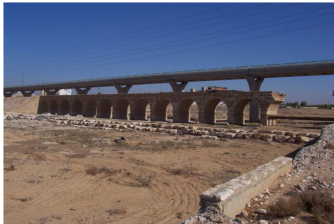
Figure 5.2. A barrel vault bridge built by the Turkish army during the First World War, Beer- Sheva Valley, Israel. Picture: Zahi Pan.
