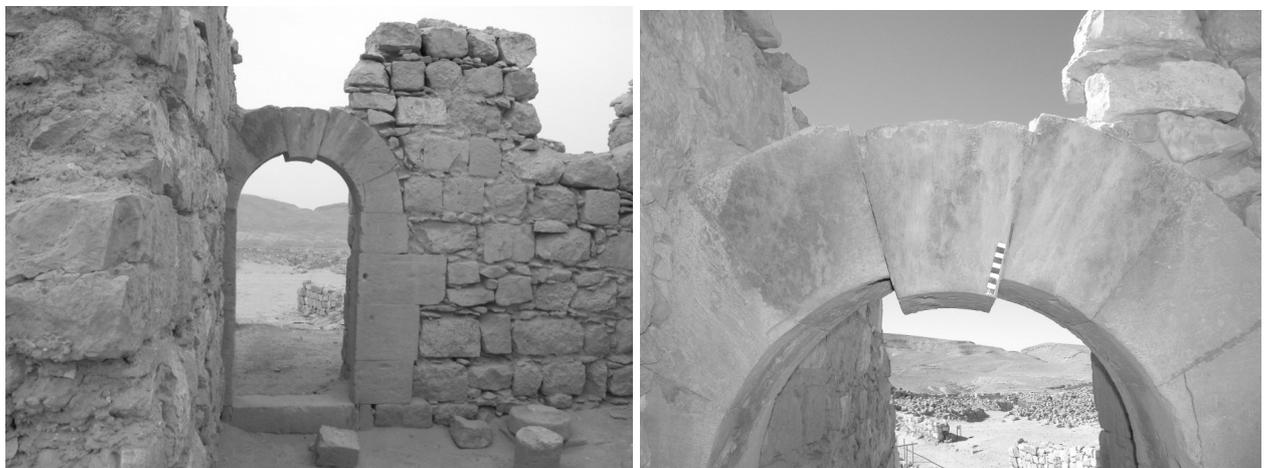
Figure 5.3. The deformed arch at Mamshit. **A.** The arch is embedded in a very heterogenic wall. **B.** The Keystone has slid 4cm downwards while the rest of the arch remained intact.
