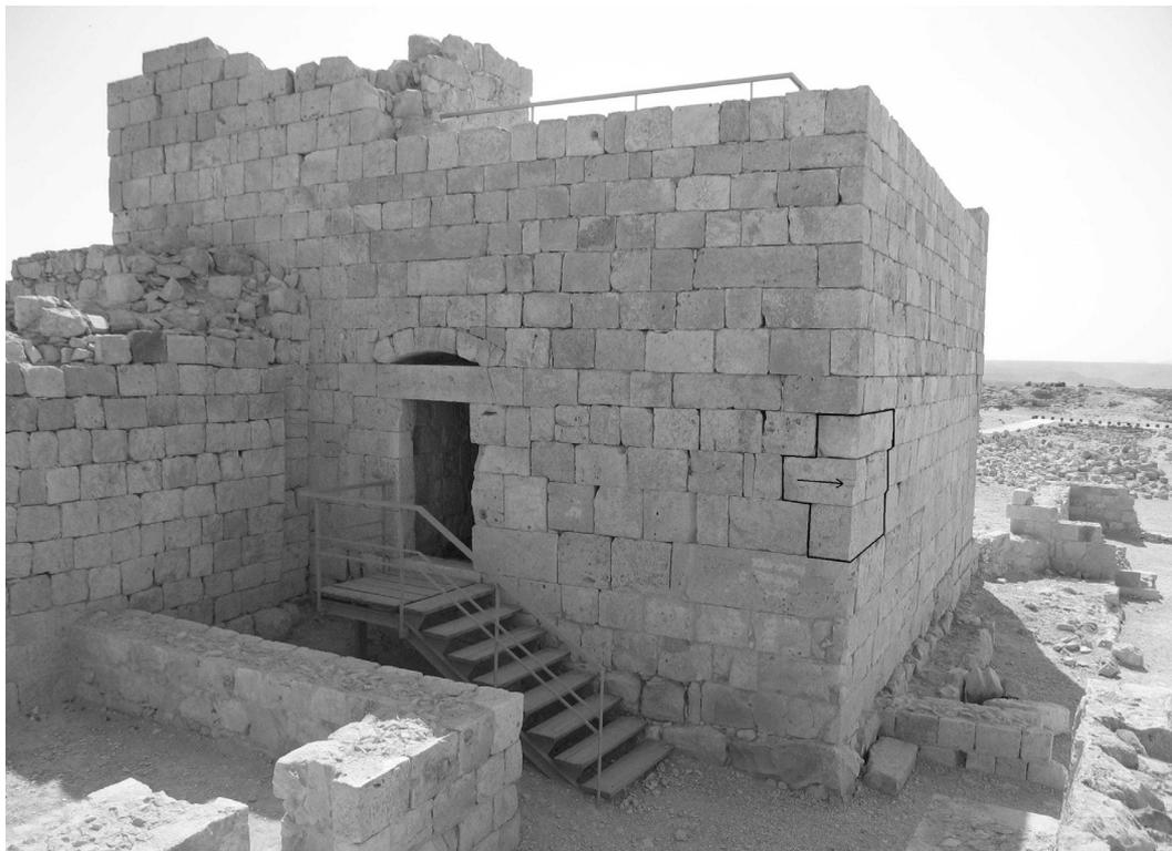
Figure 5.25. The northern wall of the roman tower at Avdat. The five corner blocks are marked and their displacement direction is displayed with an arrow.
