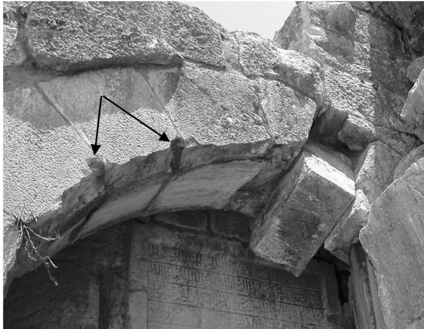
Figure 5.51. Corner chipping is seen in many of the rocks at the gate tower – an energy dissipation mechanism which can not be imitated with DDA.
