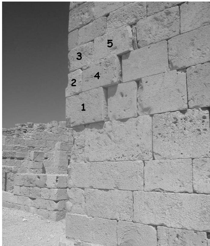
Figure 5.22. The Roman tower in Avdat, a view of the western wall. The displaced blocks are numbered for reference.
