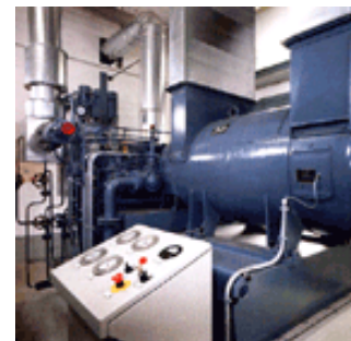
CAVIRO distillery CHP and biogas plant (Faenza, Italy)
