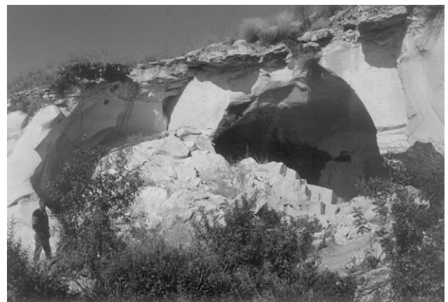
Fig. 5. A single, small span, bell-shaped cavern which collapsed during the winter of 1995 due to slippage along a pre-existing joint.
