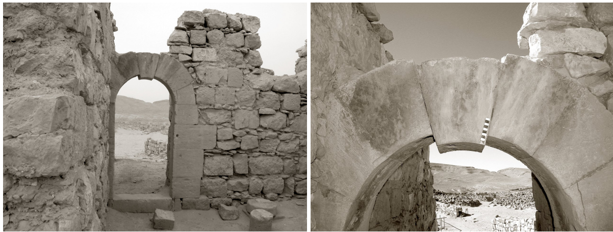
Figure 5. The damaged arch at Mamshit. A. The arch is embedded in a very heterogenic wall. B. The Keystone has slid 4cm downwards while the rest of the arch remained intact.
