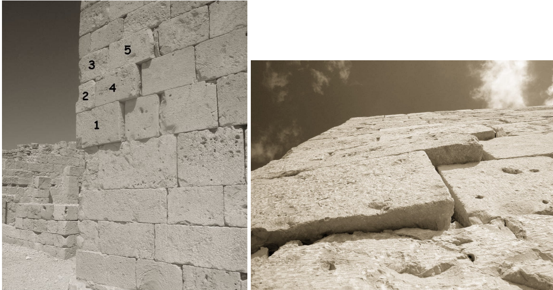
Figure 12. A. The Roman tower in Avdat, a view of the western wall. The displaced blocks are numbered for reference. B. The displaced blocks.
